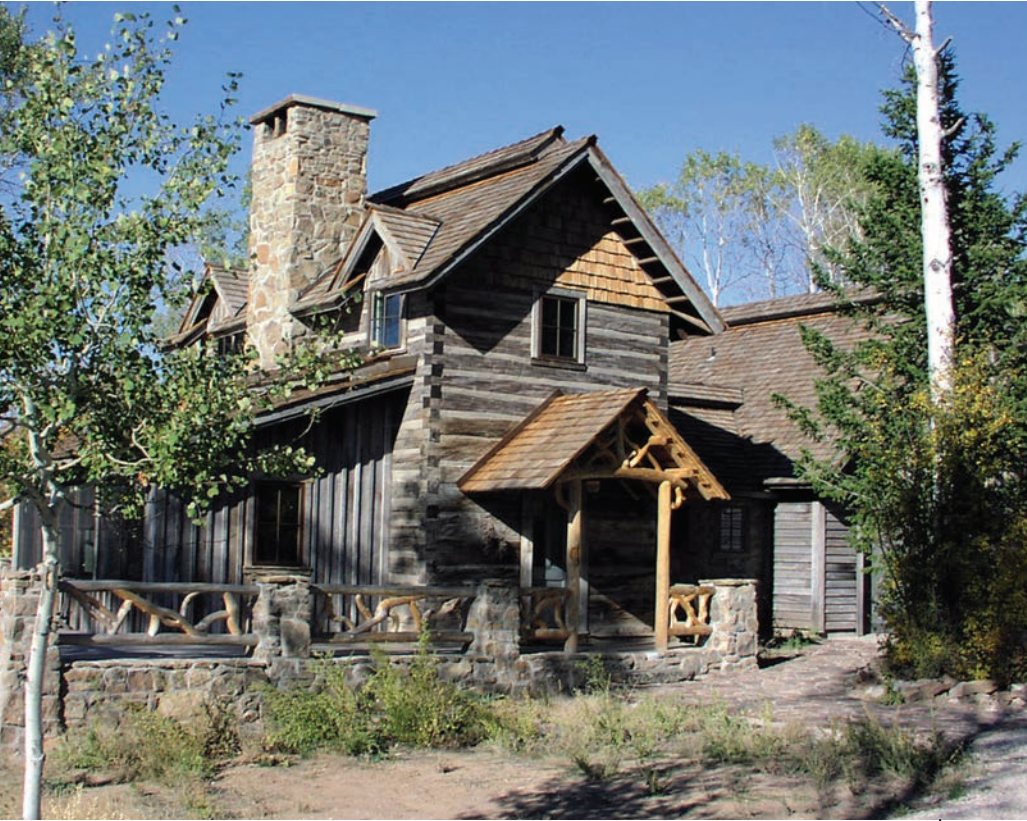
EACH PIECE OF WINTER-DAMAGED LODGEPOLE PINE WAS HAND SELECTED TO CREATE THE DESIRED LOOK.
