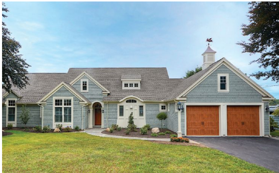
The streetside view shows how venting for the overhead rangehood in the kitchen was subtly designed into the center of the front elevation. "We worked hard to incorporate the hood into the exterior trim, and we have glass all around that. I think it worked very well," says architect Jack Kemper.
